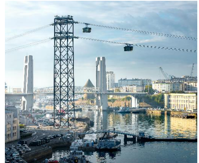
Brest Metropolis- Cable car
