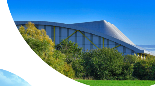
European metropolis of Lille (59) Modernization of waste sorting and treatment equipment to reduce non-recovered waste
