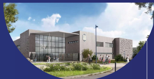
City of Toulouse (31) Construction of the Jean Zay elementary school
