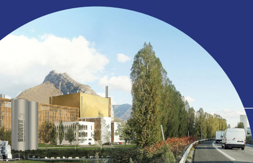
Grenoble Metropolitan area (38) Construction of a cogeneration plant
